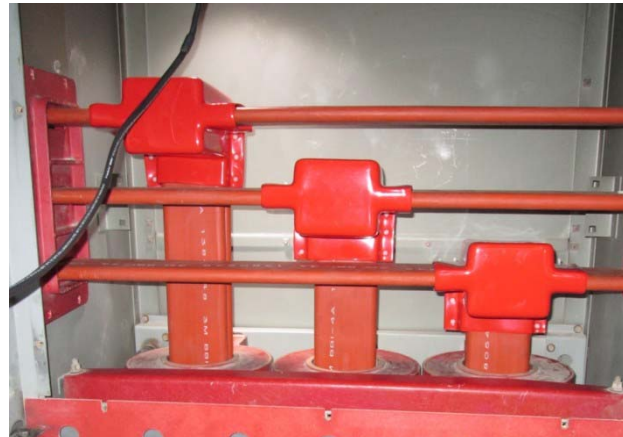
Swgr Main Bus on the refurbishment date
