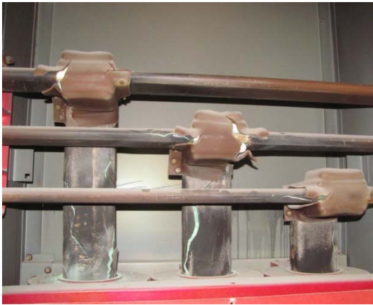
Swgr Main Bus on the inspection date
